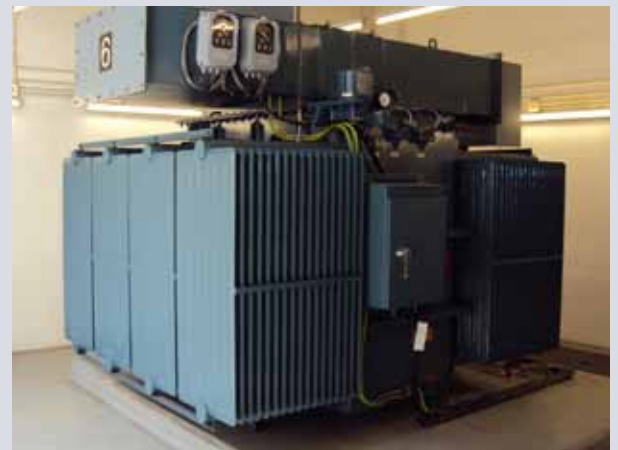
Radiator hermetically sealed type
